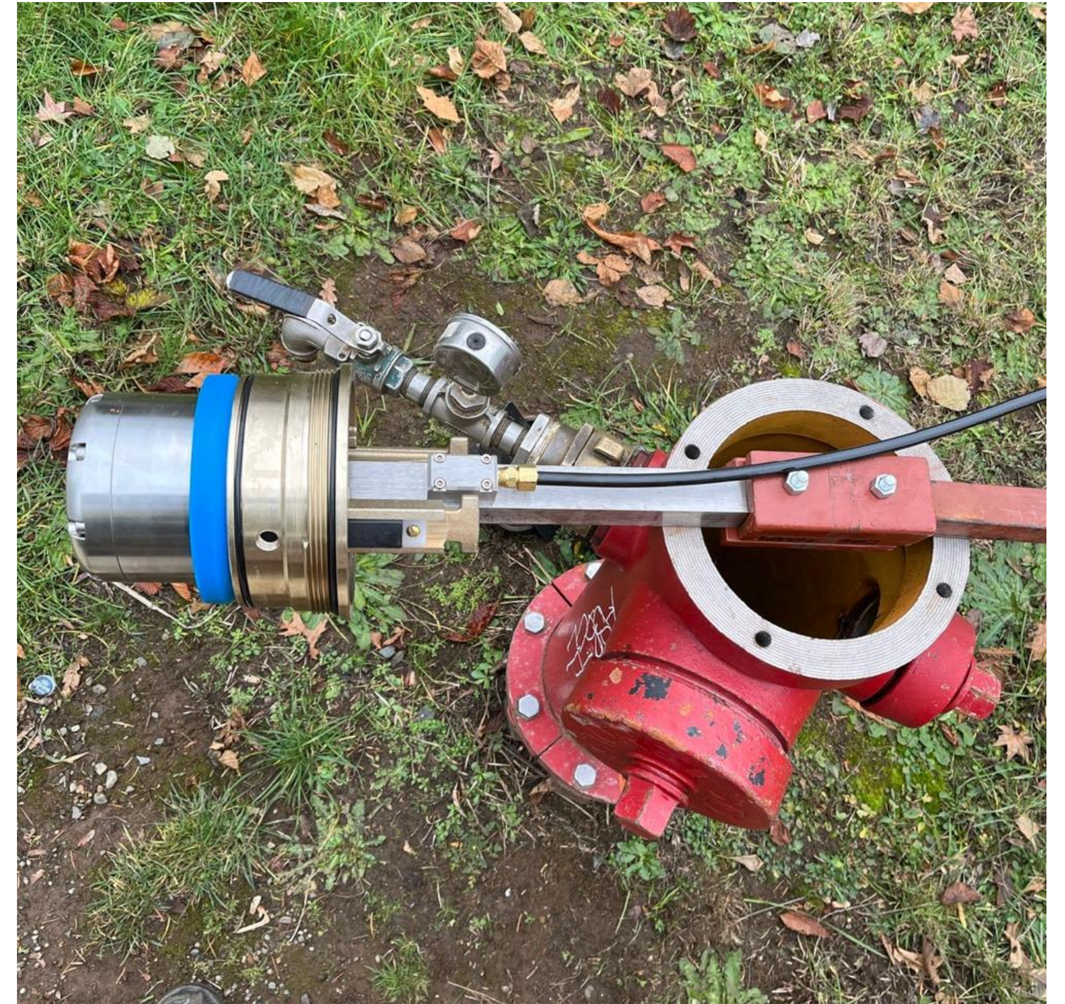
Leak Detection retrofit
