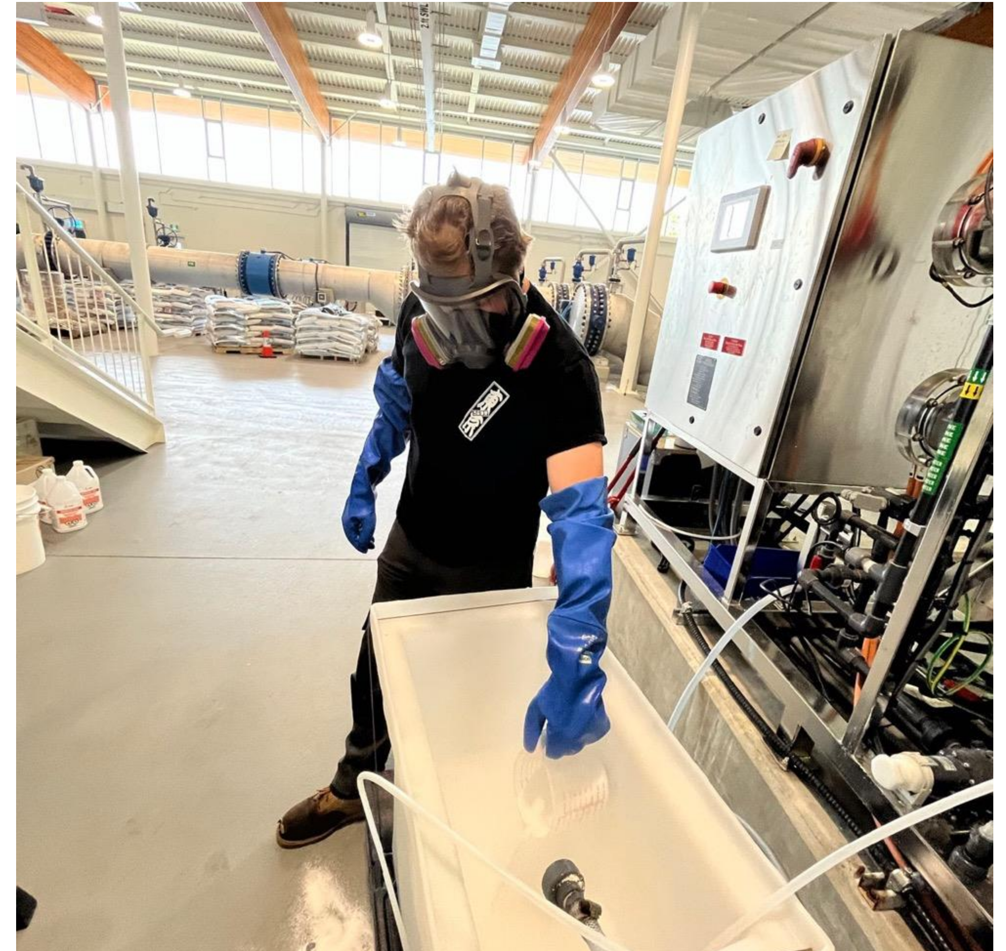
Neutralizing muriatic acid with Sodium Carbonate.
