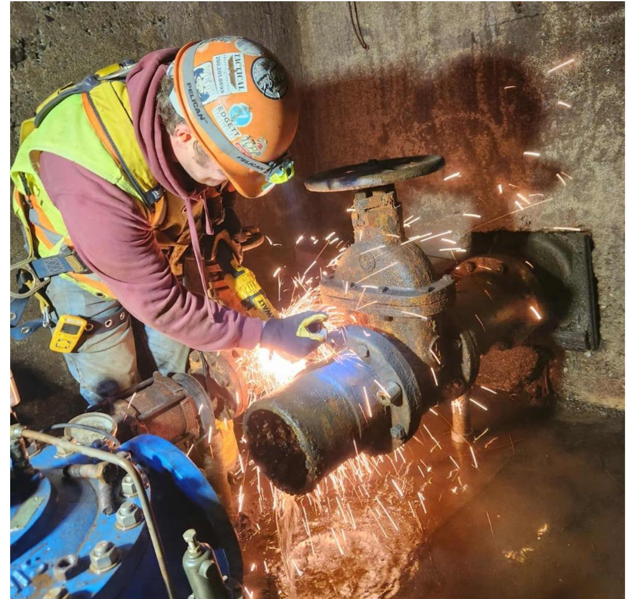
Stubborn bolts being removed to make way for PRV upgrades.
