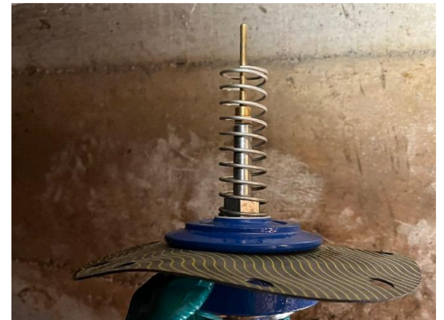
Five year Preventive Maintenance schedule has the diaphragms replaced in the main valves and pilots.
