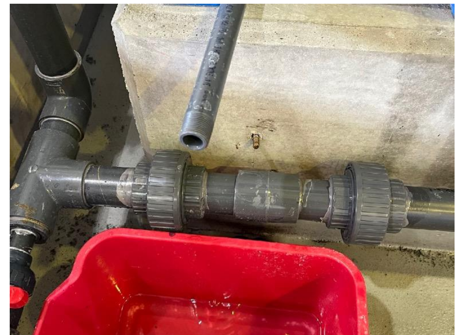
Repair on 1% hypo pump supply line.
