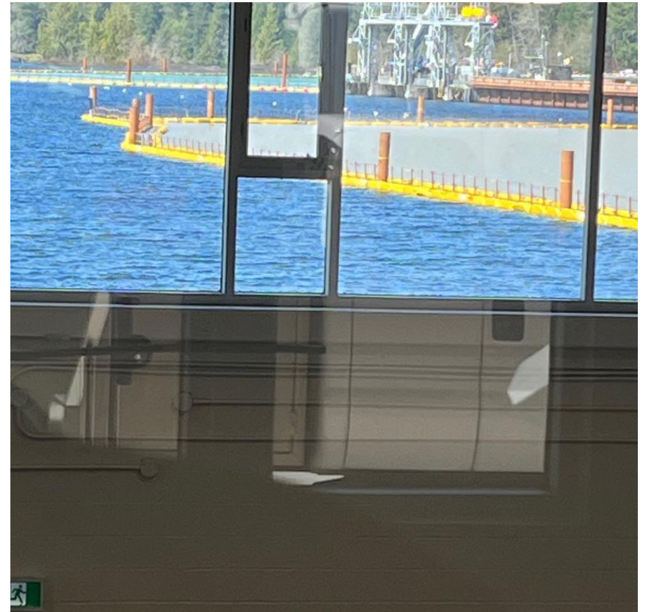
This picture highlights the proximity of turbid water being held back from John Hart lake intake.
