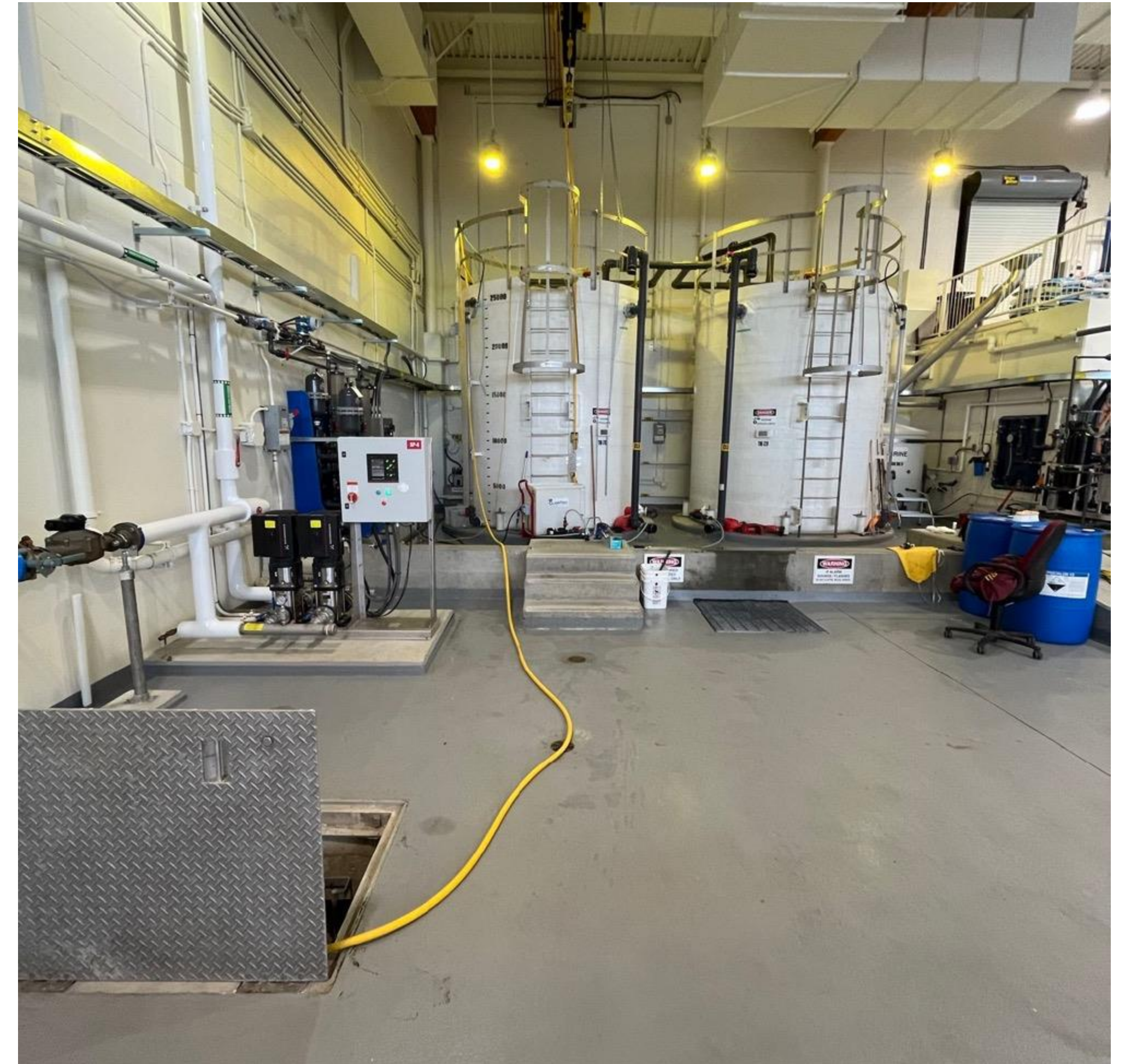
Cleaning the hypo storage tanks.
